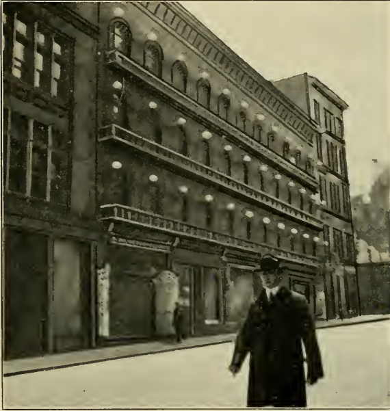
Formerly stood on Tremont Street, near Court. Demolished in June, 1903
